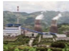
Expanded our power business in China with a conditional agreement for two coal-fired power plants in Chongqing totalling 1,620 megawatts. The plants' strategic mine-mouth location will allow for power production at a competitive cost
