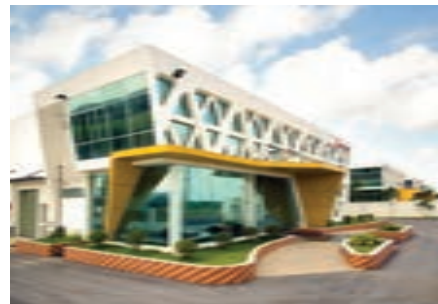
13 ready-built factories have been completed at VSIP Hai Phong with 10 factories already tenanted
