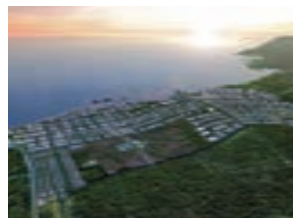
Commitments secured for land in new Kendal Industrial Park in Indonesia even before the launch of the project
